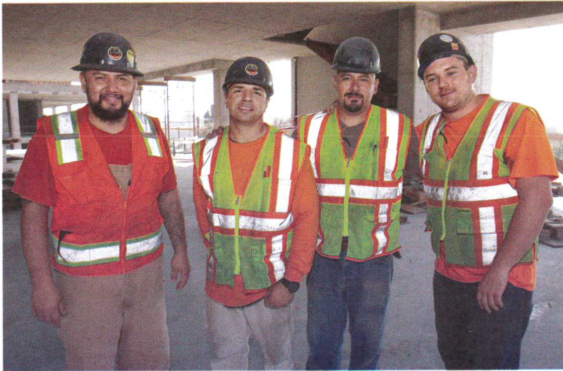
(l-r) From UA Local 709 Sprinkler Fitters, Marc Espinoza, Mark Hanna, Ricardo Campos and Juventino Herrera. "It's been a really well-kept job site and really well-coordinated," says Hanna, an apprentice.
